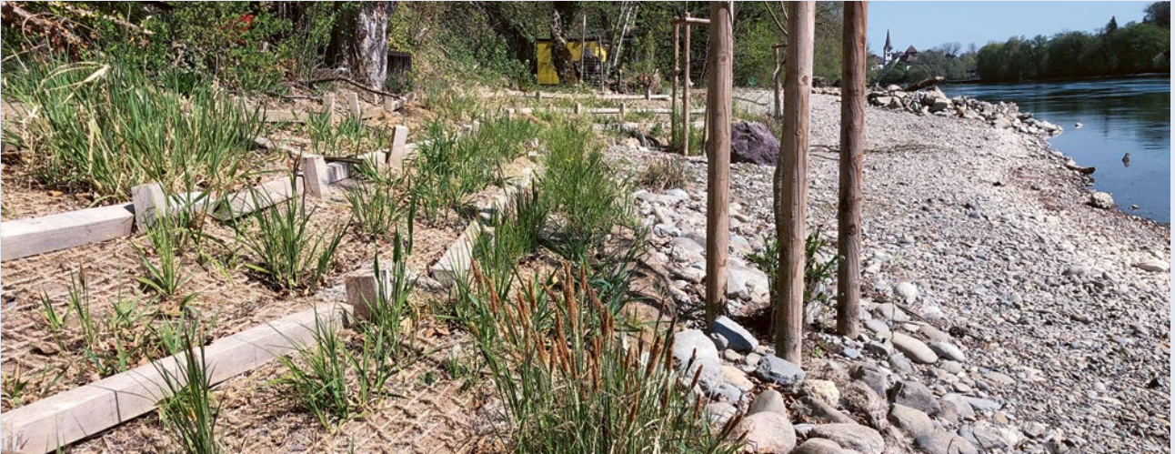
Coconut fibre and sheep's wool mats were planted with native species such as reed canary grass and various sedges to provide near-natural protection for the river's banks (photo: SH Power).
