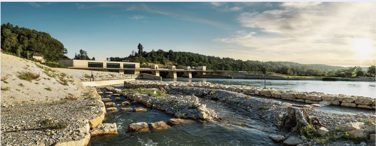
The refurbished Hagneck power plant integrates harmoniously with its natural environment. (Photo: BKW)
