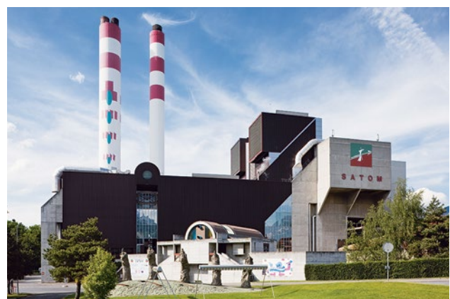
The Monthey waste incineration plant of SATOM AG was the first plant to be awarded under the Climate Charter. It plans to obtain naturemade resources star certification in 2018. (Photo: SATOM AG)
