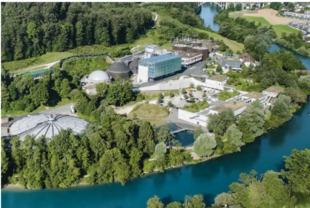
The arabern waste water treatment plant in Berne has been producing naturemade star-certified biogas since 2009. (Photo: arabern)
