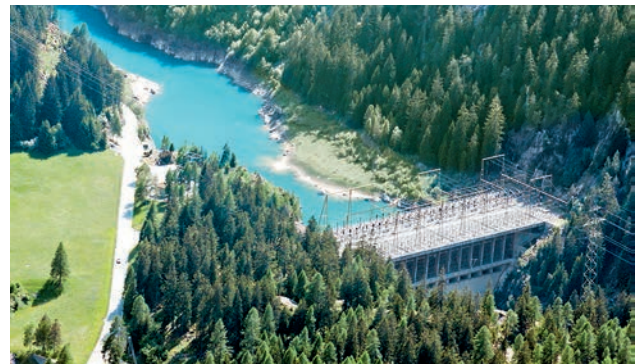
The Hinterrhein AG power plants completed the required residual flow upgrades in 2014. (Photo of the naturemade basic-certified Bärenburg power plant: Kraftwerke Hinterrhein AG)
